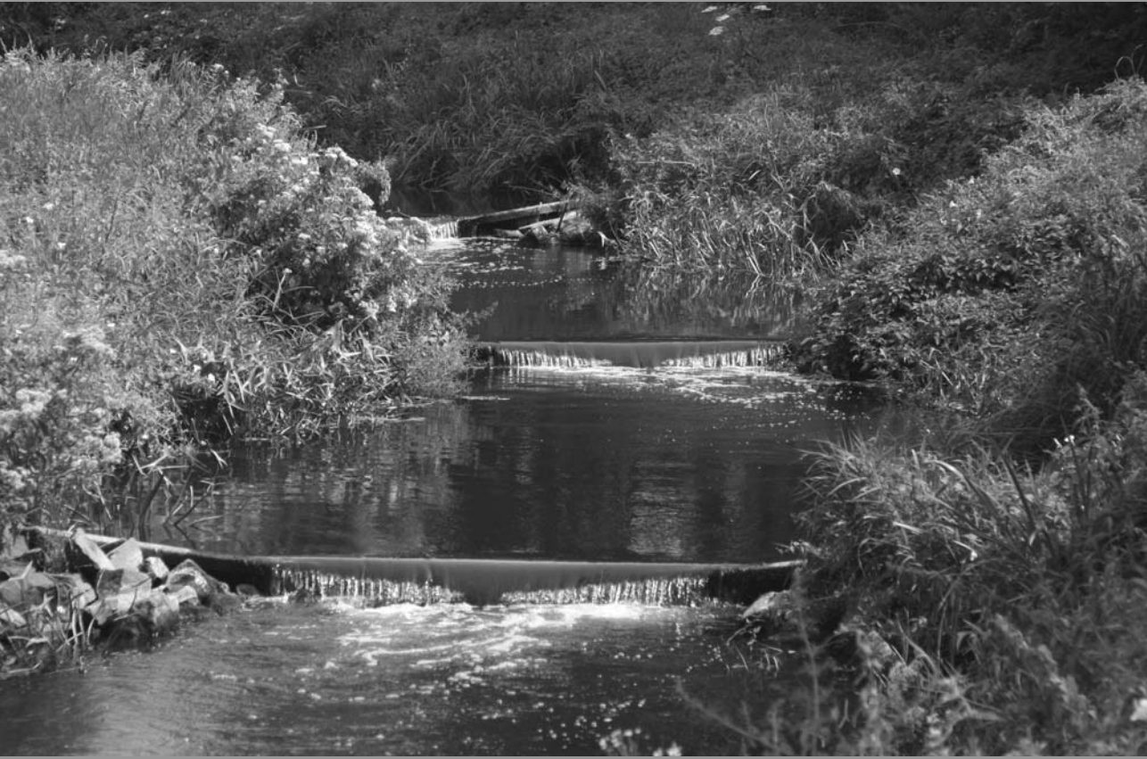
Fishway in the Vecht / Vistrap in de Overijsselse Vecht
